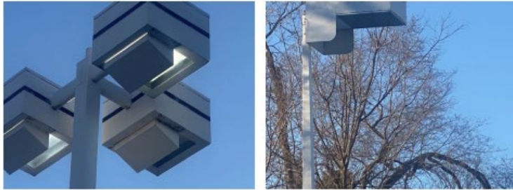
Exhibit 3: Cutoffs and baffles used at Bredemann Ford to reduce light pollution to neighbors.
